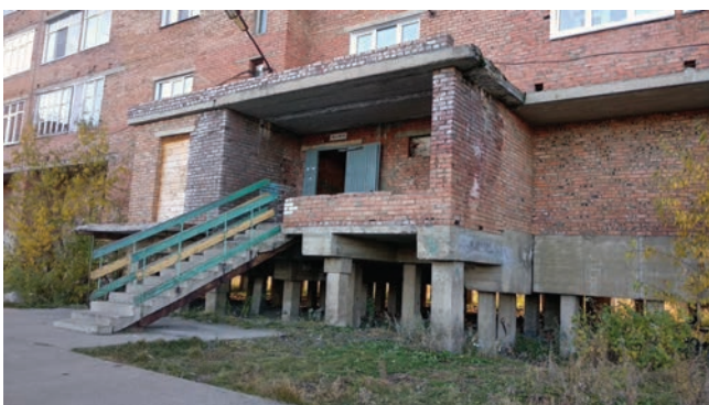
Figure 8.1a. The elevation of buildings (and other infrastructure) onto pillars allows for a ventilated layer between the structure and the ground, which helps protect against permafrost degradation: Igarka, Russia. Photo: Nadezhda Zamyatina
